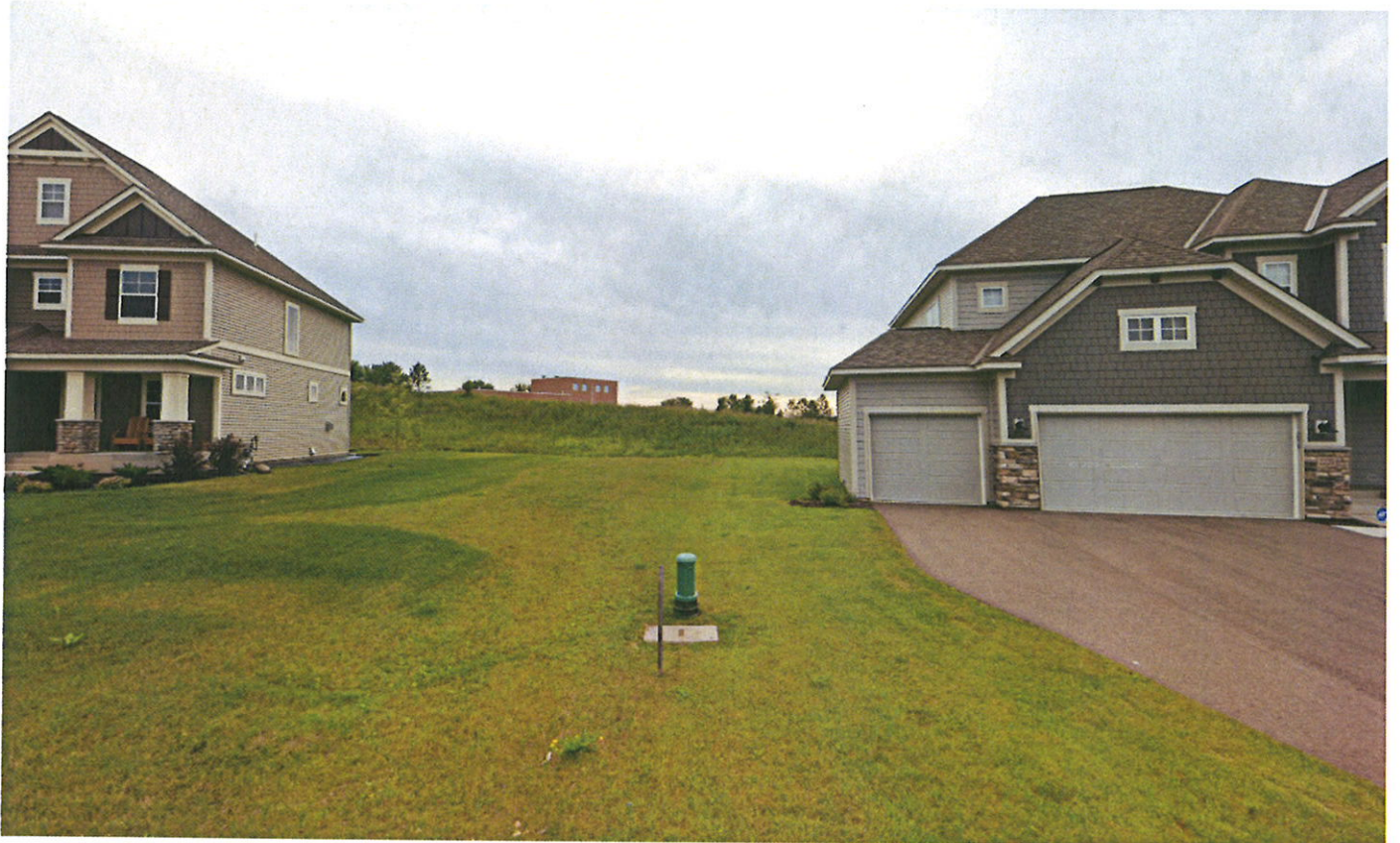
Comparable neighborhood view of Water Treatment Facility
