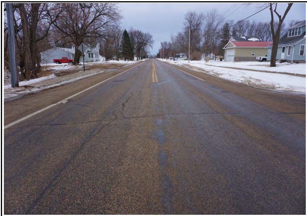
Looking South along S. Agency Street from Maywood Avenue
