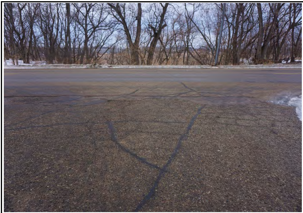
Looking East at S. Agency Street & Maywood Avenue Intersection
