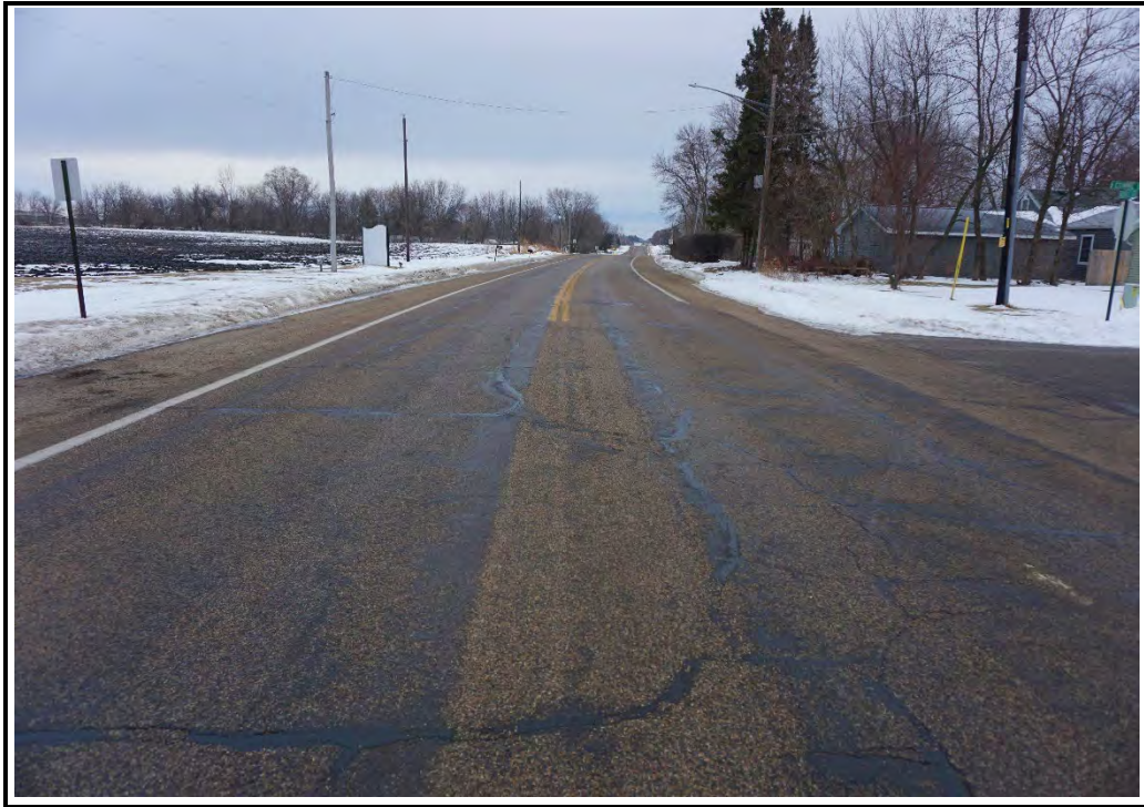
Looking South along S. Agency Street from Connie Lane
