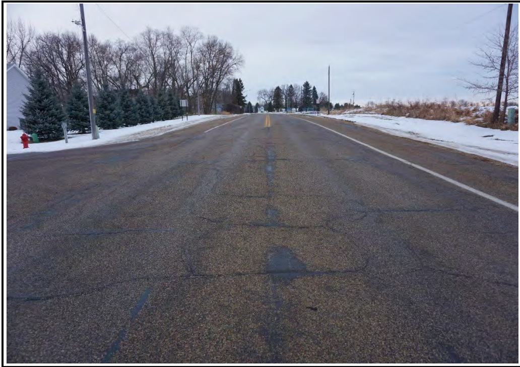
Looking North along S. Agency Street from Thomas Drive
