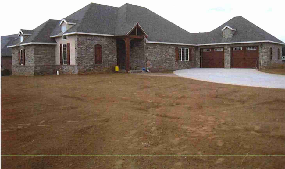
Final grade (left) is properly sloped away from the home and ready for permanent vegetation.
