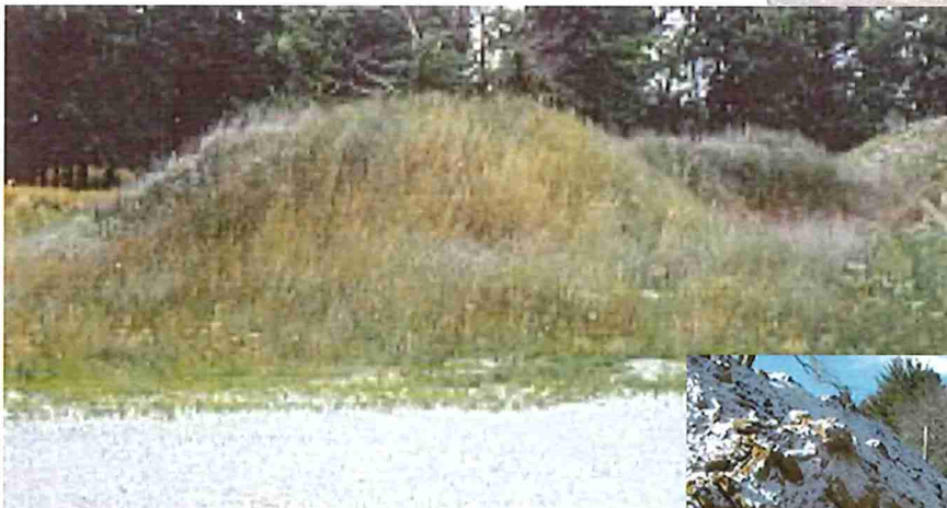
Stockpiles that remain for periods longer than 14 days must be seeded as photo to the left shows.
