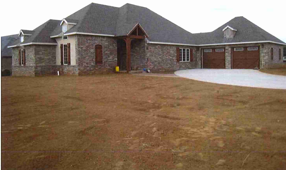
Final grade (left) is properly sloped away from the home and ready for permanent vegetation.
